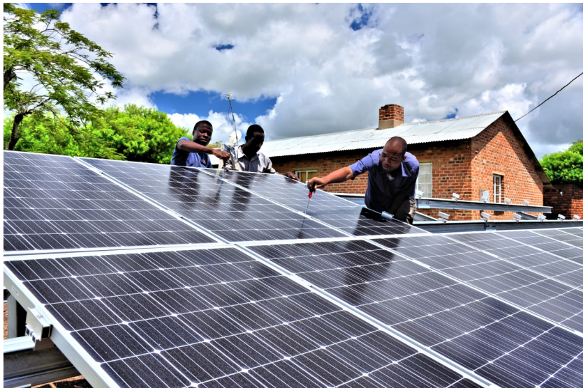
Mounting the 36 solar panels that are the heart of the solar power facility that provides electricity for the hatchery.
