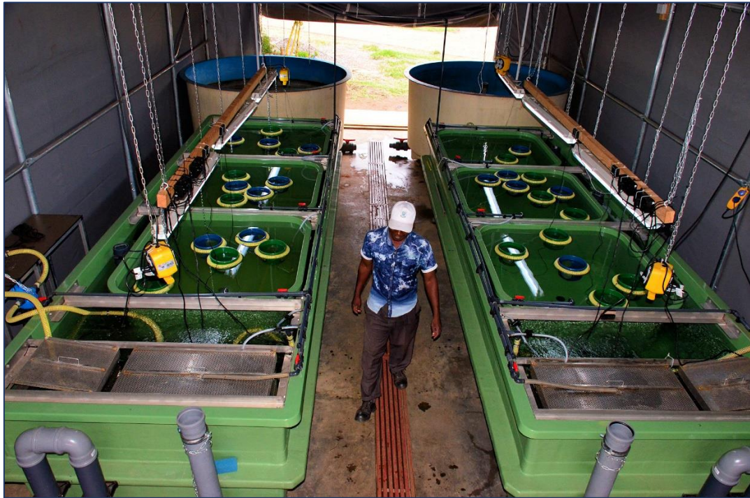
Fig. 7: Hatchery ready to operate. The circular tanks in the background can be used as store tanks for water exchange. They can always be filled when well-water is available and sufficient solar power is available to operate the water pump at the well.
